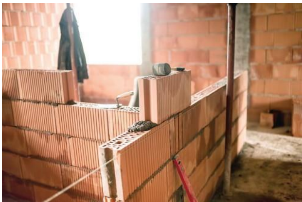
Fig. 31. ceramic partition wall
