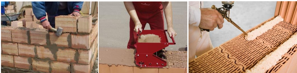
Fig. 20. conventional mortar, thin mortar and adhesive bond technology
