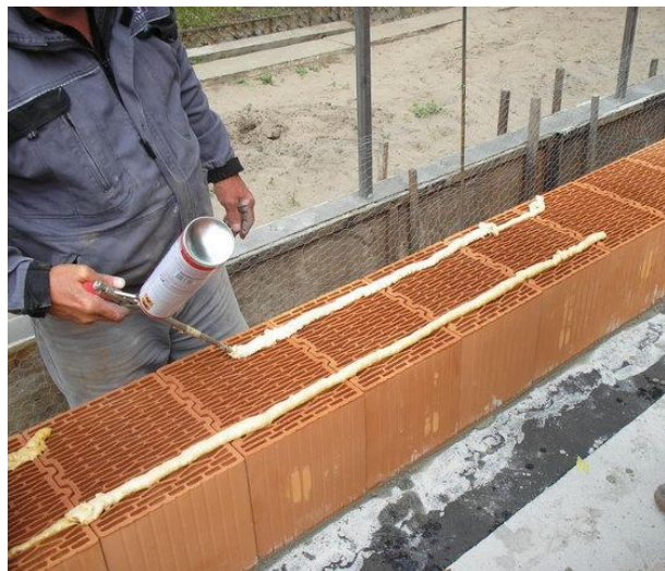
Fig. 24. adhesive foam technology
