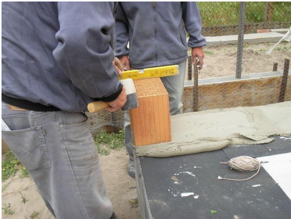
Fig. 21. setting of the corner brick
