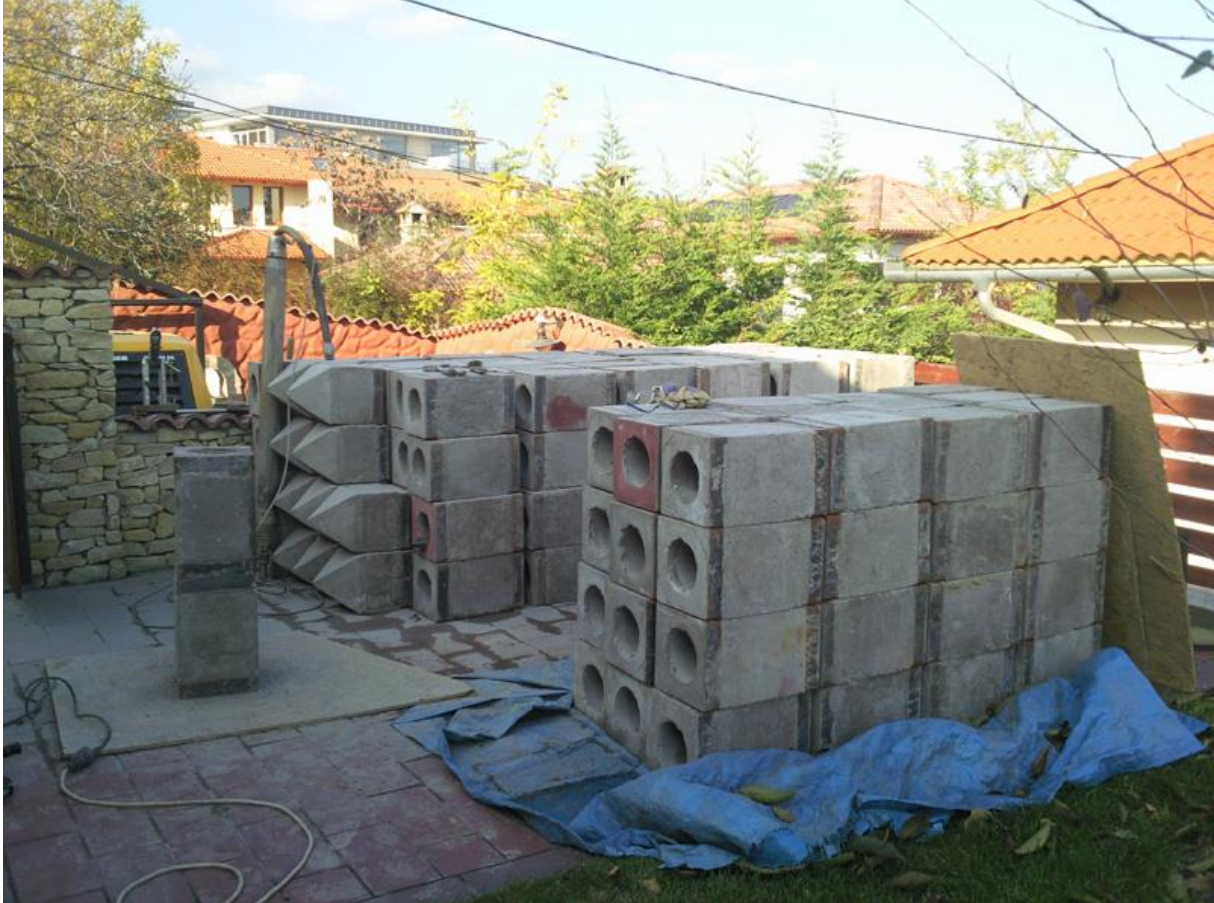
Fig. 71. Mega pile elements
