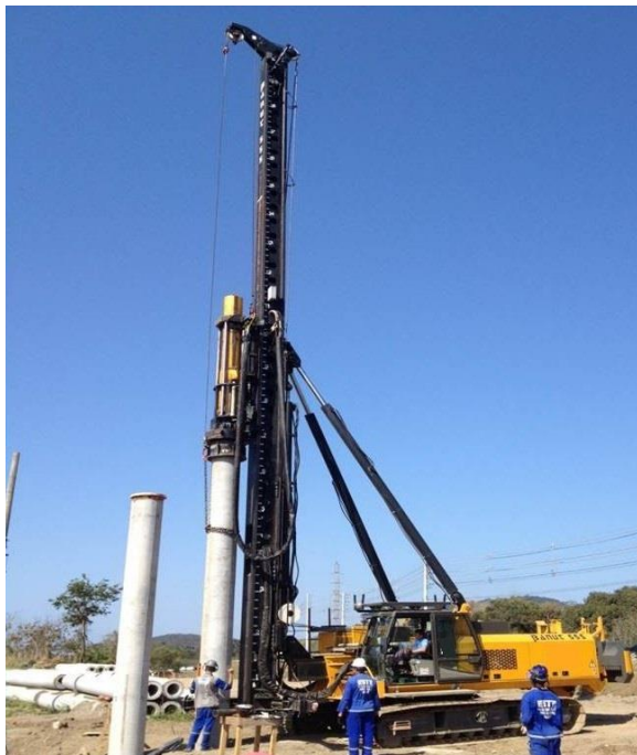
Fig. 51. Pile driving
