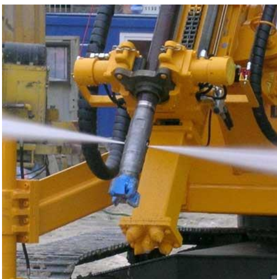
Fig. 69. Jet grouting
