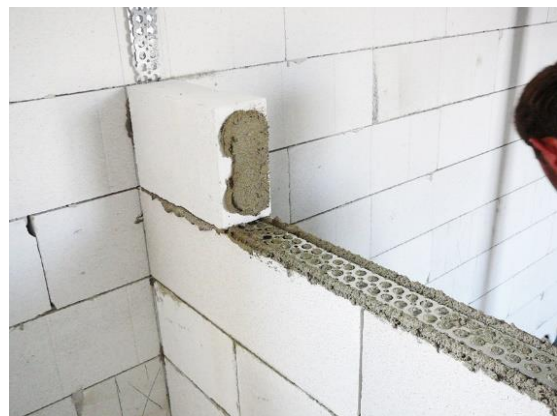
Fig. 30. aerated concrete partition wall
