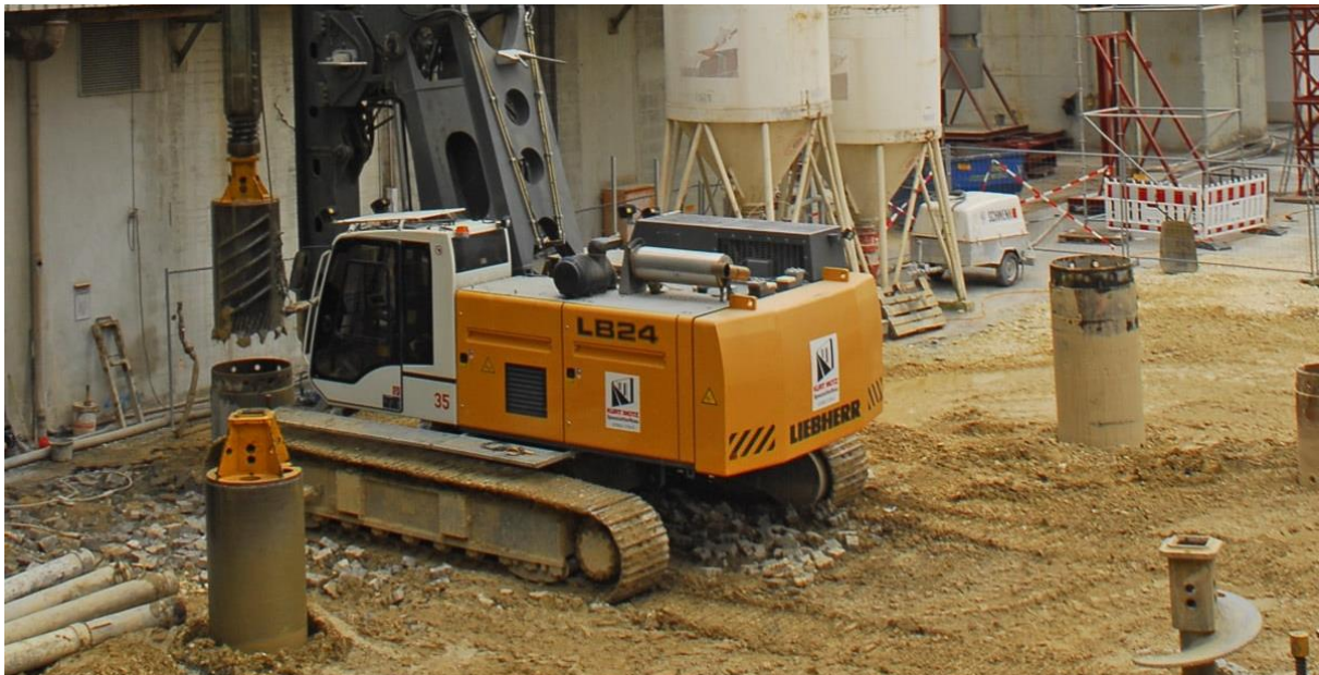
Fig. 54. Pile boring
