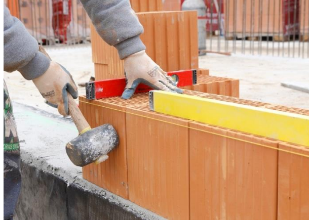
Fig. 22. laying of the first course
