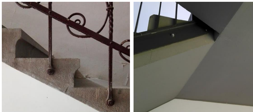
Fig. 86. Stone and reinforced concrete stairs
